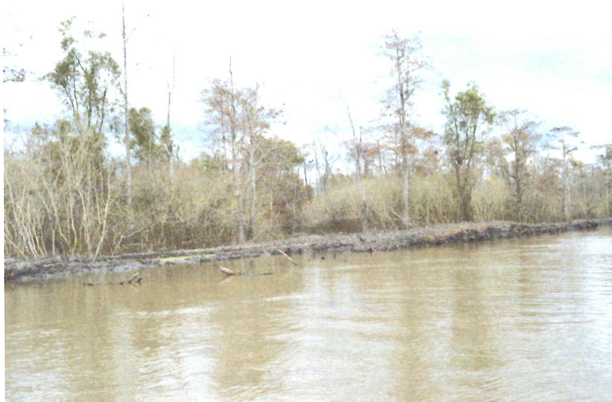
Figure E: This photo was taken by Dean Wilson during the monitoring trip in the Basin on December 7, 2018. This photo was taken at the following approximate coordinates: 30.08608056, -91.39916667. This photo depicts a waterway dammed by pipeline construction in this area.
