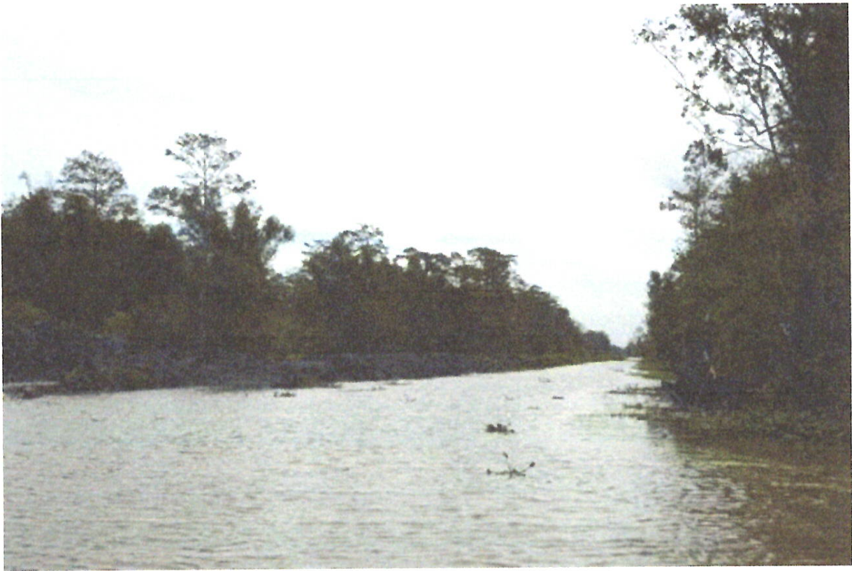
Unnamed bayou dam
